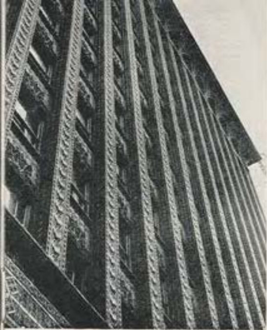
The Guaranty Building. Sullivan
